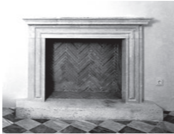
22b. Isti nakon obnove (snimila N. Vasić, Hrvatski restauratorski zavod). Fireplace after renovation (photo by N. Vasić, Croatian Conservation Institute)
