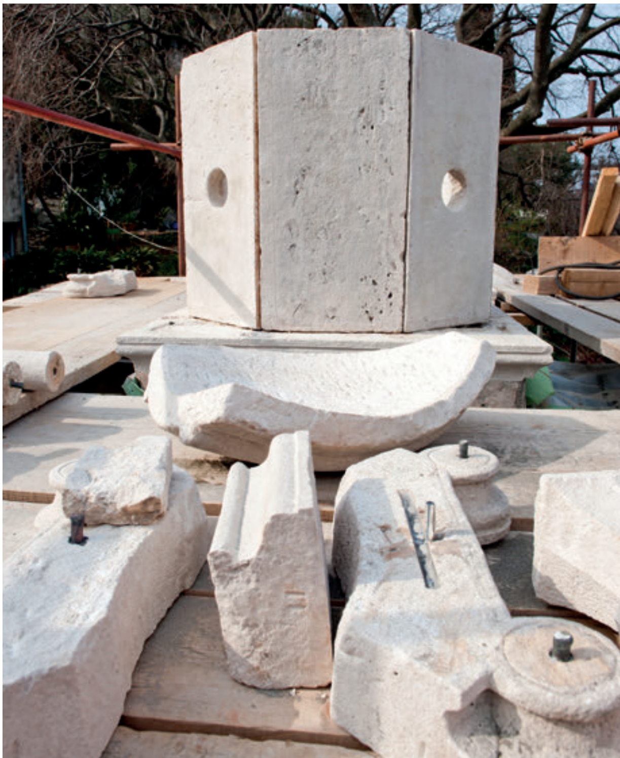
26. Rastavljeni dijelovi kupole kapele tijekom restauratorskih radova (snimila K. Gavrilica, Hrvatski restauratorski zavod). Dismantled sections of the chapel dome, in the course of conservation (photo by K. Gavrilica, Croatian Conservation Institute)
