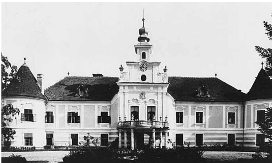
Jugozapadno pročelje nakon dogradnje altane / Southwest front after the altana was added
