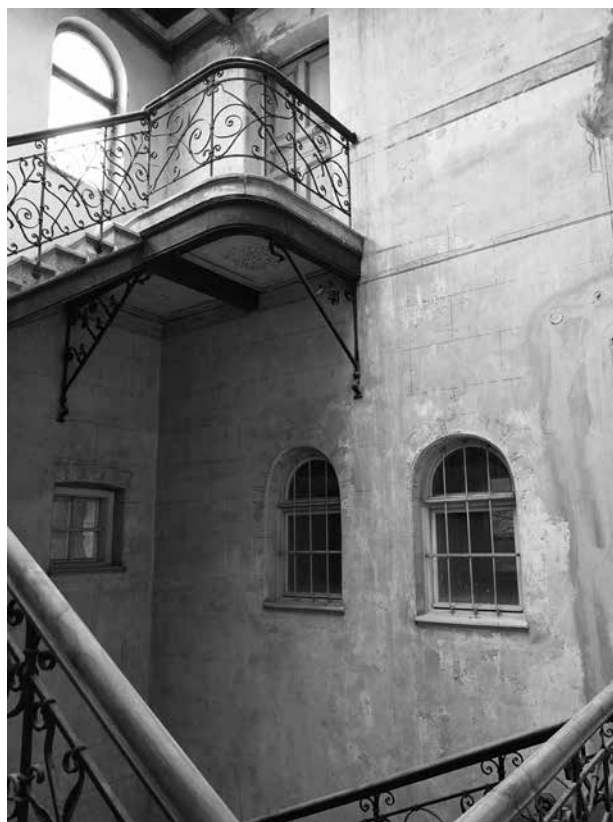
Oslik zida i stubište na drugom katu zgrade u Žerjavićevoj 4 (foto: D. Damjanović, 15. 7. 2013.) / Wall painting and staircase on the second floor of the building in 4 Žerjavića street
