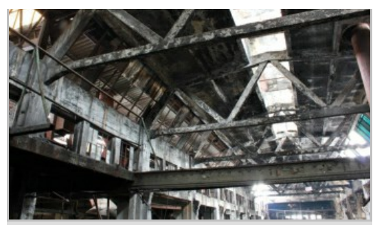
Picture 2: Main factory building roof construction Photo: authors' photo archives, 2011.
