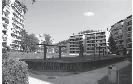
Figure 9 The Pilot Action Target Area Before Renovation
