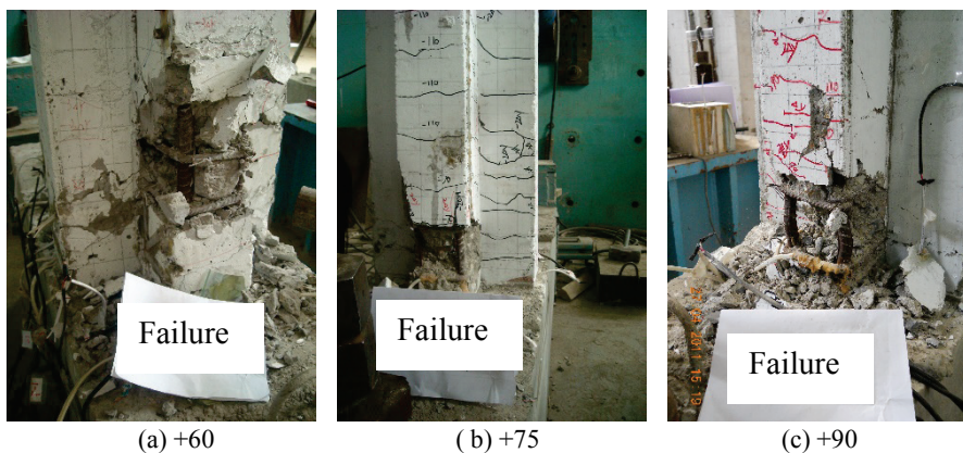
Figure 4 Failure mode of cross-shaped columns
