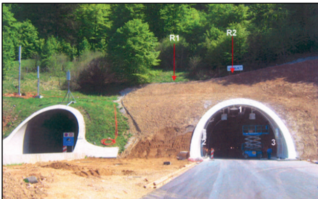
Figure 5 The Sleme Tunnel portal with marked positions of the measuring points 1, 2, 3, R1 and R2 of the right tube
