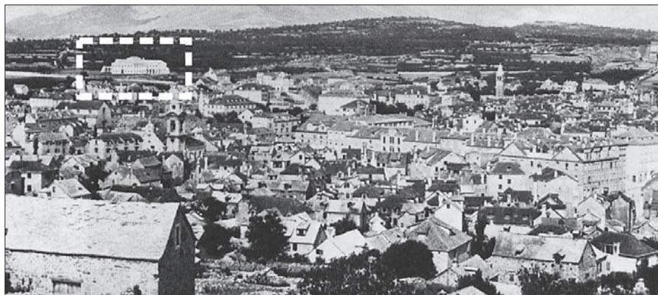
FIG. 4. VIEW OF SPLIT FROM MARJAN HILL, THE FIRST BUILDING OF CHARITABLE HOUSING FOUNDATION MARTINIS-MARCHI FROM 1871 DOMINATES THE VACANT AREA OUTSIDE THE HISTORICAL BOUNDARIES, PHOTOGRAPH FROM 1870S
