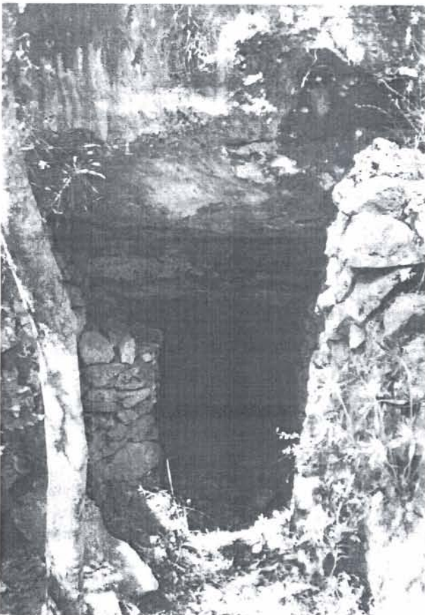
Sl. 11. Ulaz u rudnik Škrip na otoku Braču. Lijevo je dio ulaza u niskop obložen suhozidom od jalovih karbonatnih stijena Fig. 11. Entry into a mine Škrip on the Island of Brač. On the left is a part of the entrance into the incline lined with dry stone walling of carbonate rocks
