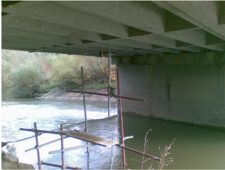
Fig. 10. Scaffold under the bridge.
