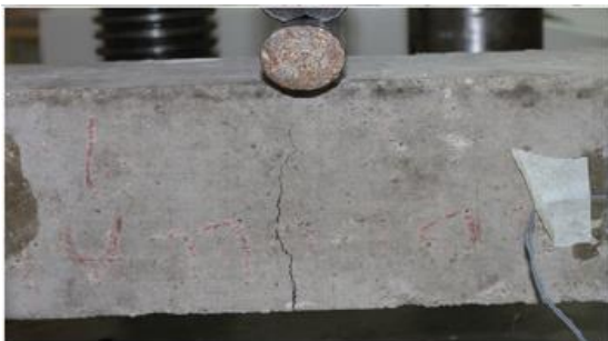
Figure 2. Failure mode for beam B2, content 1.0% steel fibers [7].
