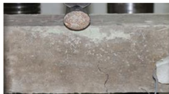
Figure 1. Failure mode for beam B2, non-fiber reinforced concrete [7].
