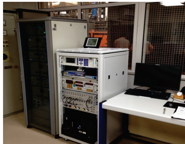
Figure 2 High voltage test laboratory
