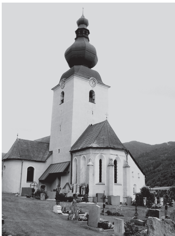
19. Župna crkva u St. Georgen ob Judenburg (Štajerska), očuvan primjer tipa 'Chorturm'. / Parish church at St. Georgen ob Judenburg (Štajerska), preserved church of the "Chorturm," type.
