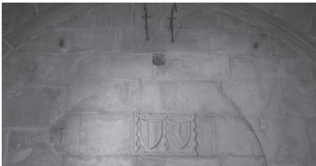
Kapela sv. Jeronima, zapadni zid s tragom zazidanog okula i grbovima patricijskih rodova Vitturi i Casotti / St. Jerome's Chapel, West wall with the trace of the original oculus and coats of arms of Vitturi and Casotti families
