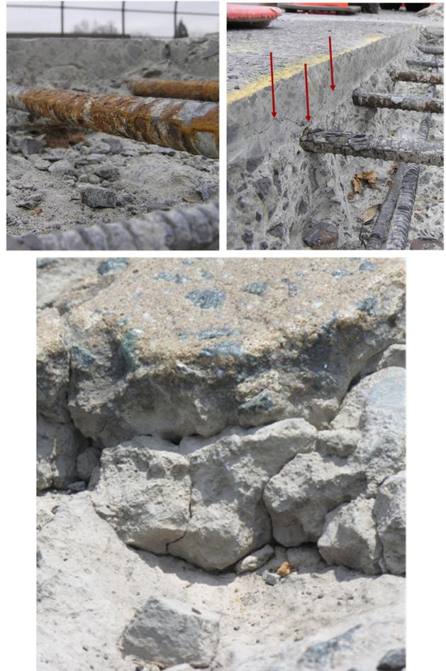
**Figure 1** Typical concrete bridge deck deterioration and damage: rebar corrosion (left), delamination (middle), and deck spalling (right).
