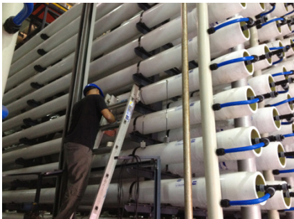
Figure 2. Installation of AE system on FRP vessels.
