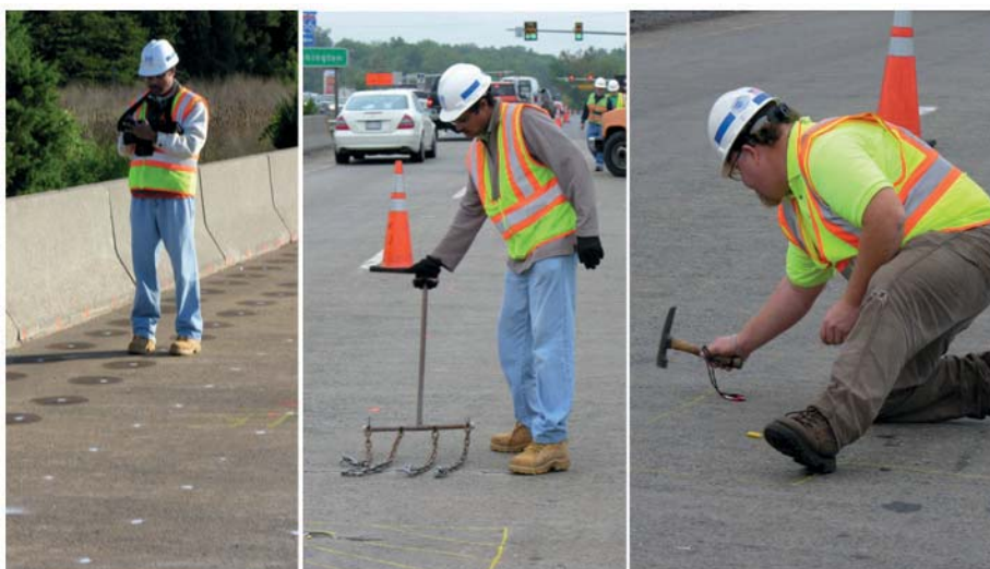
Figure 1. Visual inspection (left), chain-drag (middle) and hammer sounding (right) of a bridge deck.
