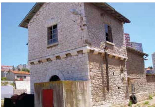
16 Željeznički kolodvor, vodosprema (foto: I. Šprljan) Railway station, water reservoir (photo: I. Šprljan)
