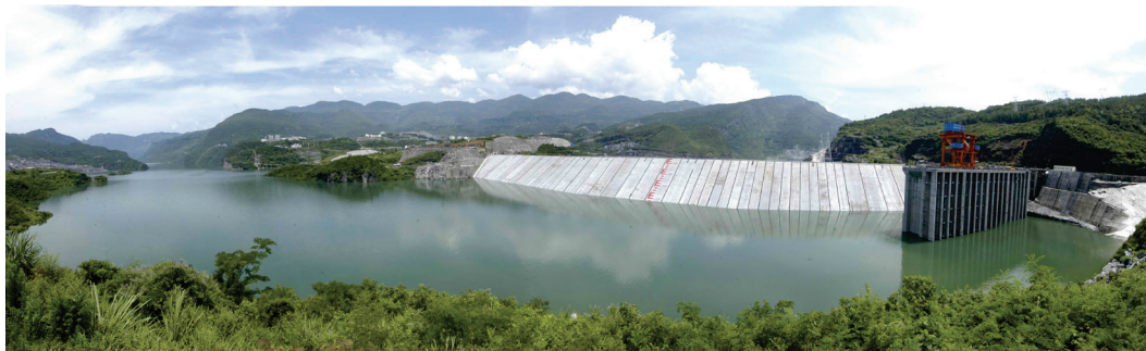
Figure 2 A general view of the Shuibuya CFRD
