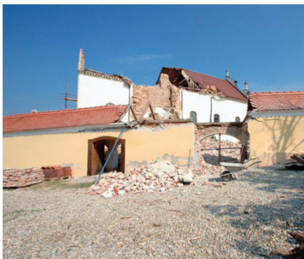
5. Lopatinec, župna crkva sv. Jurja mučenika snimljena nakon rušenja zvonika i svoda nad svetištem (snimila N. Vasić 2008., fototeka HRZ-a) Lopatinec, parish church of St. George the Martyr photographed after the belfry and the sanctuary vault collapsed (photo by N. Vasić, 2008, Croatian Conservation Institute Photo Archive)
