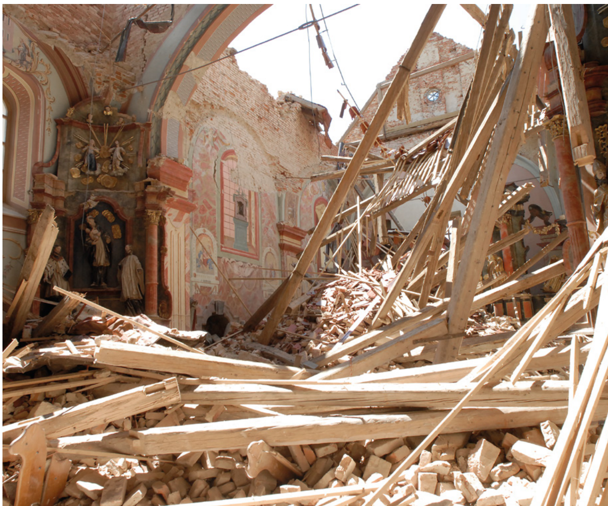
4. Lopatinec, župna crkva sv. Jurja mučenika, pogled na svetište nakon rušenja zvonika i svoda (snimila N. Vasić 2008., fototeka HRZ-a) Lopatinec, parish church of St. George the Martyr, view of the sanctuary after the belfry and the vault collapsed (photo by N. Vasić, 2008, Croatian Conservation Institute Photo Archive)
