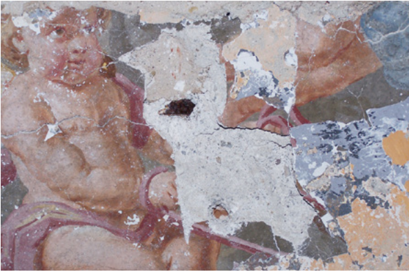
8. Detalj fragmenta s oštećenjima žbukanih slojeva. Slojevi su mjestimično odvojeni od opečnog nosioca (snimila V. Šulić, 2007.) Detail of the fragment with visible injuries to the plaster layers and its detachment from the brickwork (photo by V. Šulić, 2007)
