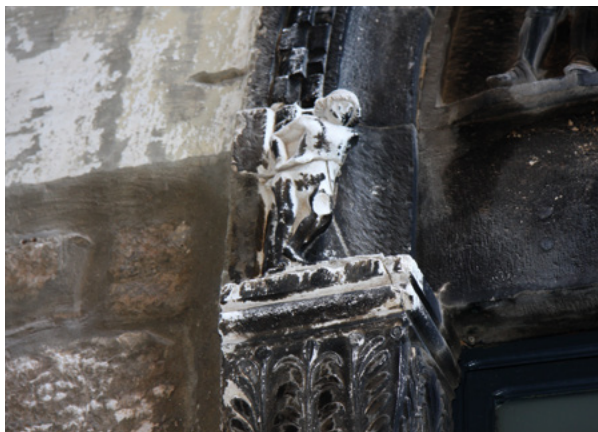
1. Crna kora, ili crna skrama? Portal palače u Ulici Jurja Barakovića u Šibeniku, detalj (snimila K. Hraste, 2014.) Black crust, or black encrustation? Portal of the palace at Juraj Branković St. in Šibenik, detail (photo by K. Hraste, 2014)
