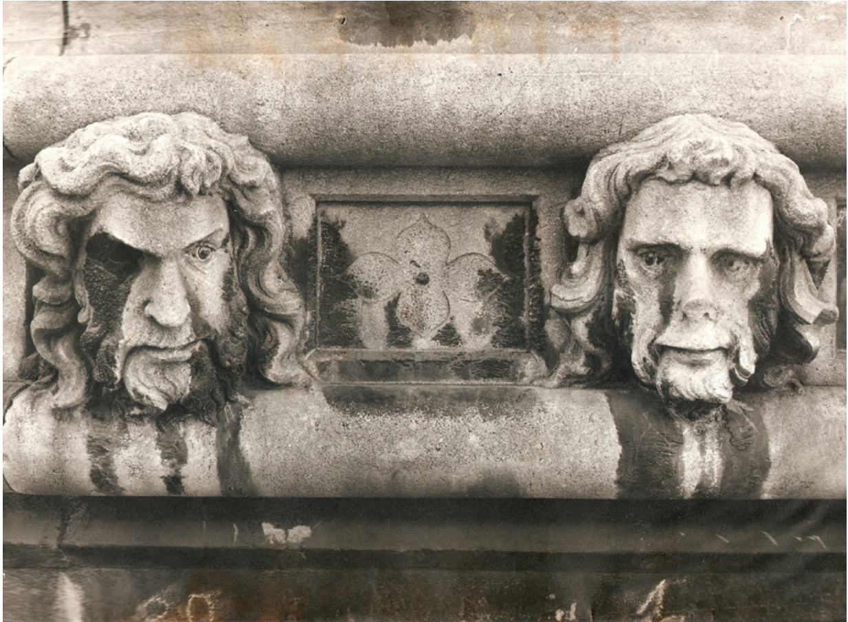
8. Crne kore i tamne prevlake ili crne kore i sive patine? (snimio H. Malinar) Black crusts and dark coating or black crusts and grey patina? (photo by H. Malinar)
