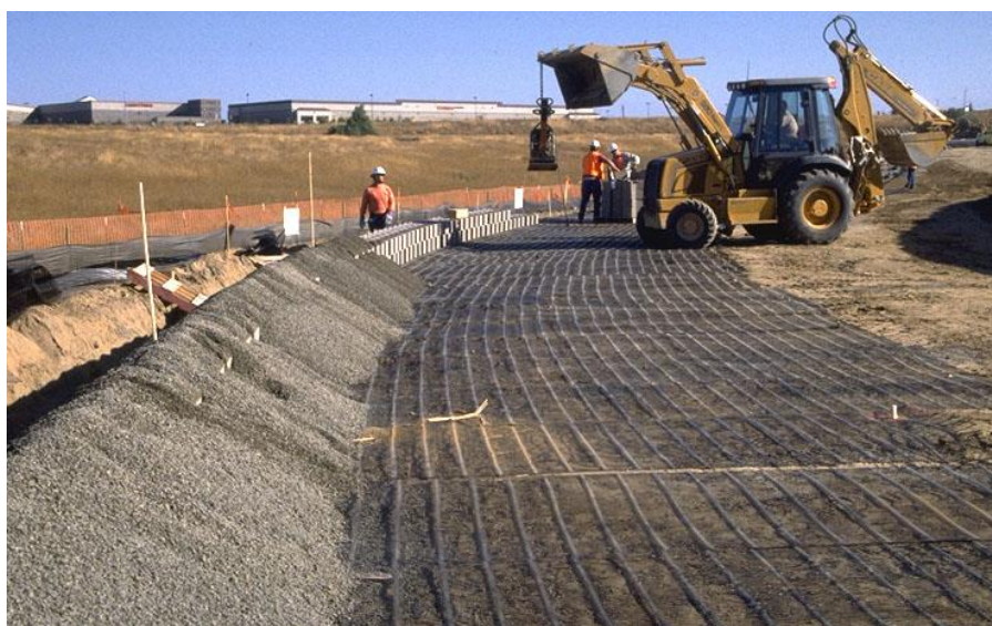
Figure 11 Placing the fill material between geogrids (image source: http://research.engineering.ucdavis.edu/gpa/wp-content/uploads/sites/43/2015/02/Rein.-Soil-Wall-P3-Labeled.jpg )
