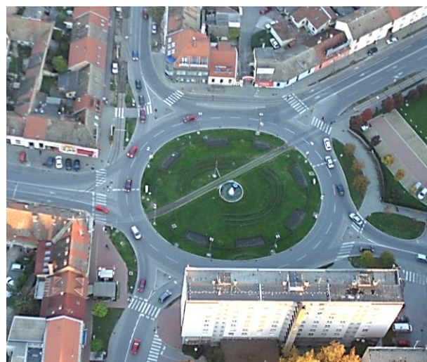
Figure 1 Aerial view of the Đakovština roundabout
