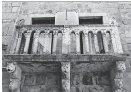
SL. 9. BALKON KNEŽEVA DVORA U RABU S KONZOLAMA OBLIKOVANIM KAO DVOSTRUKE LAVLJE GLAVE FIG. 9. BALCONY OF THE DUCAL PALACE IN RAB WITH CONSOLES SHAPED AS PAIRS OF LION HEADS
