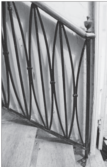
SL. 19. DETALJ OGRADE OD KOVANOGA ŽELJEZA IZ 19. STOLJEĆA U KUĆI PETROVSKI FIG. 19. DETAIL OF THE WROUGHT-IRON RAILING DATING FROM THE NINETEENTH CENTURY IN THE PETROVSKI HOUSE
