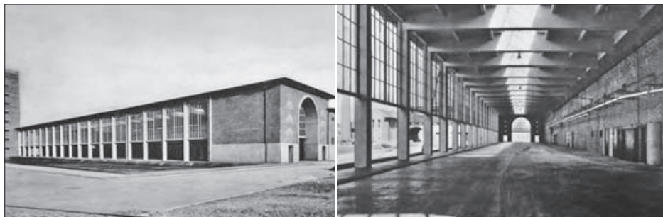
SL. 9. OTPREMNA HALA, IZVORNO STANJE FIG. 9. SHIPPING ROOM, ORIGINAL CONDITION
