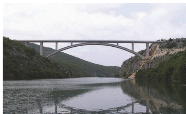
Figure 1. Aerial view of Cetina River bridge
