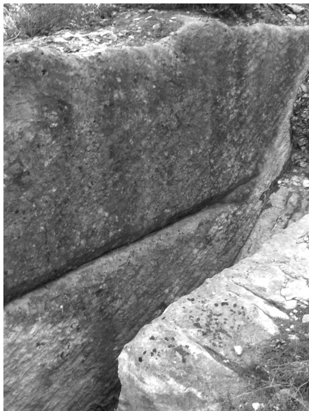
Fig. 10. Toolmarks on a quarry-face in the Plate district
