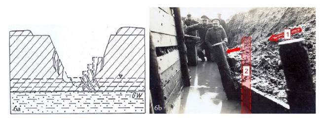
**Figure 6** Profile of a trench (6a) dug in clay soil with displayed deformations on the trench wall (**Bülow et al., 1938**) and a trench dug in clay (6b) on which a sliding phenomenon is visible (1 – sliding direction, 2 – initial position of the stake) (**Photographer not identified; observations and marks on the photo were made by the author of the article**)
