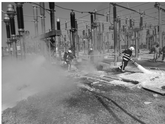
Slika 2. Gašenje požara energetskih kabela pjenom Figure 2. Extinguishing a fire on power cables with foam
