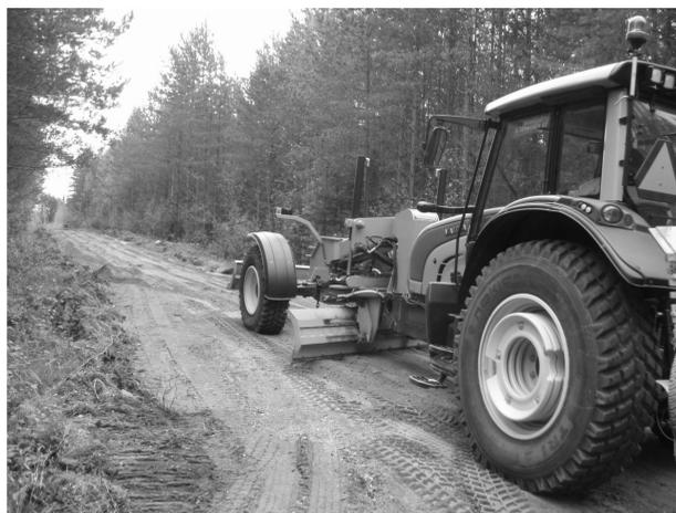
**Fig. 3** A road grader was used to shape the road surface and mix the ash and aggregate
