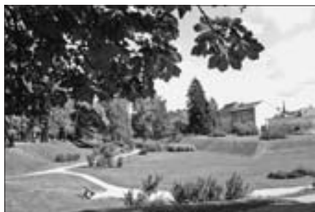
SL. 7. PROSTOR OPKOPA ISPRED BANSKOGA BASTIONA POČETKOM 21. ST. FIG. 7 MOAT IN FRONT OF BANSKI BASTION, EARLY 21 ST C.
