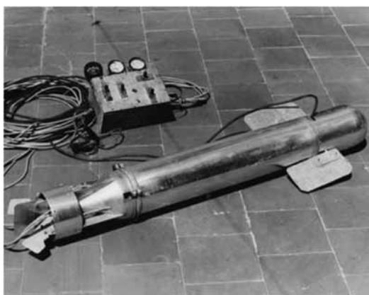
Figure 1. First ROV POODLE by Dimitri Rebikoff, built in 1953.
