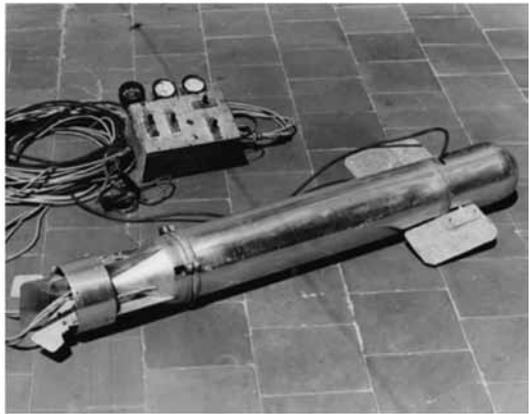
*Figure 1. First ROV POODLE by Dimitri Rebikoff, built in 1953.*
