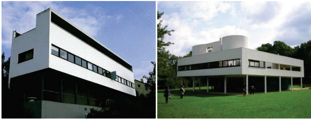
Figure 7 House in Stuttgart, Germany, 1927 (Le Corbusier) and Villa Savoye, Poissy, France, 1929 (Le Corbusier)
