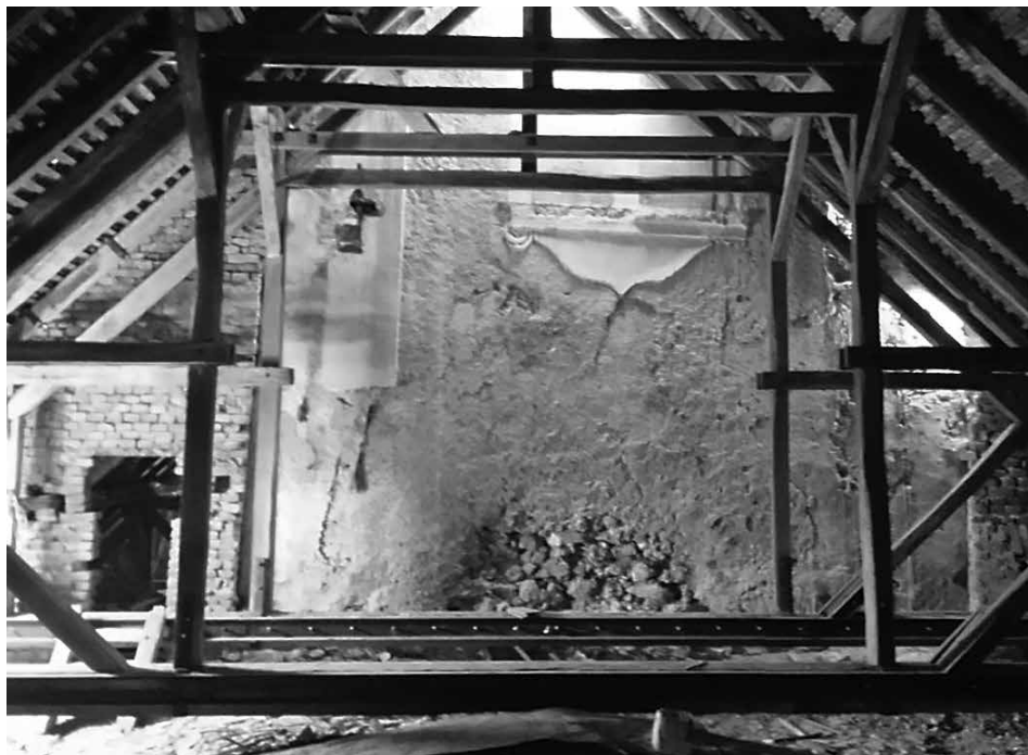
3. Tragovi žbukane bifore i pilastra na istočnom pročelju zvonika, danas zaklonjenom krovijem iznad lađe (foto: M. Strugar) / Traces of the plastered blind two-bay window and a pilaster on the belltower's east façade, now enclosed by the roof of the church's nave (photo: M. Strugar)
