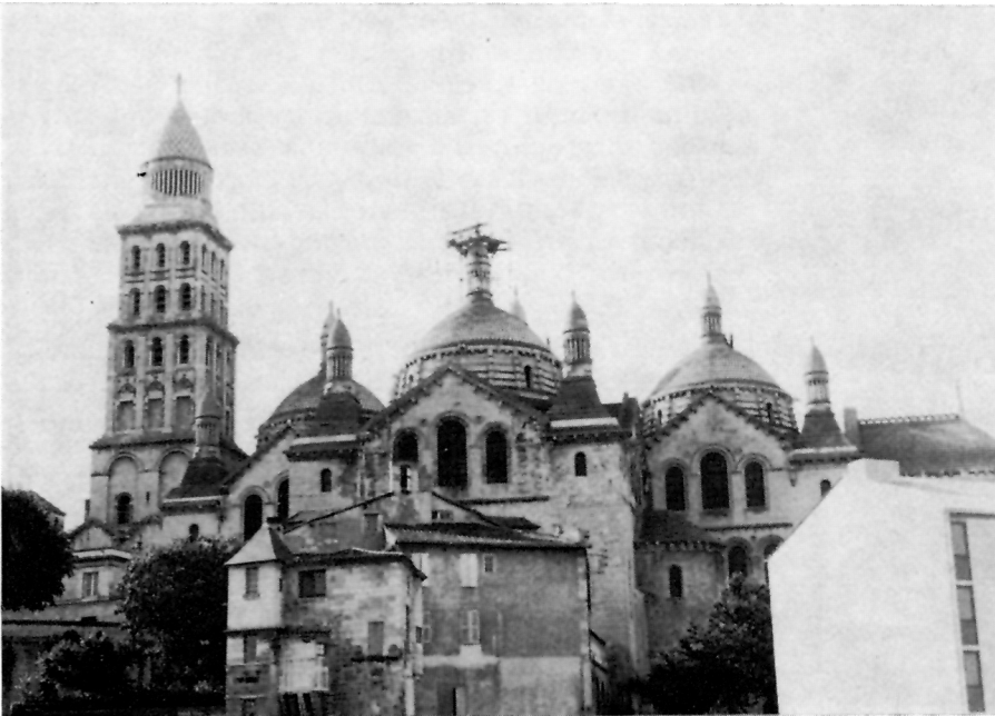
1 PERIGUEUX, St. Front — Exterior (from the South)
