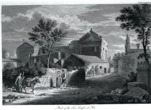
Sl. 5 Pogled na začelje dvaju hramova s prikazom nadograđene krovne konstrukcije s dimnjakom na Augustovom hramu (Stuart-Revett 1816.). Fig. 5 A view of the back wall of the two temples, with a depiction showing the roof structure and chimney which have been added onto the Temple of Augustus (Stuart-Revett 1816).
