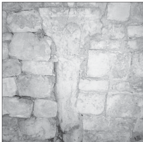
SL. 14. DETALJ ZAZIDANOGA TRIJEMA U PRIZEMLJU FIG. 14. WALLED-IN PORCH ON THE GROUND LEVEL, DETAIL
