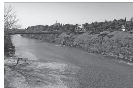
FIG. 12 VIEW UPON THE MORAČA RIVER WEST BANK SL. 12. POGLED NA ZAPADNU OBALU RIJEKE MORAČE
