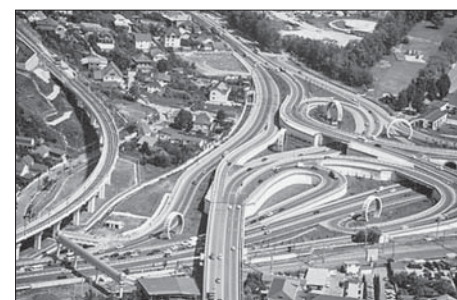
FIG. 12 ONE OF THE NEW MOTORWAY JUNCTION OUTSIDE SOCHI
