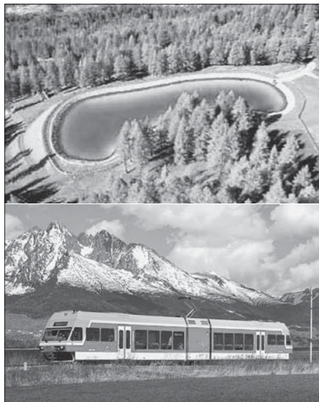
FIG. 14 RESERVOIR FOR ARTIFICIAL SNOW MAKING IN THE ALPS
