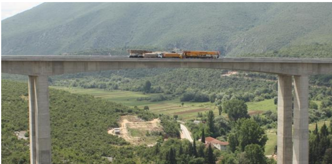
Figure 4 Test load on the bridge [6]
