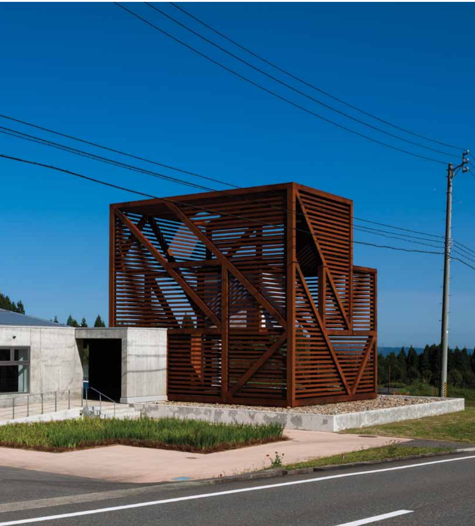
Juxtaposition of the Clubhouse (left) and Lantern/Lighthouse Pavilion (right)
