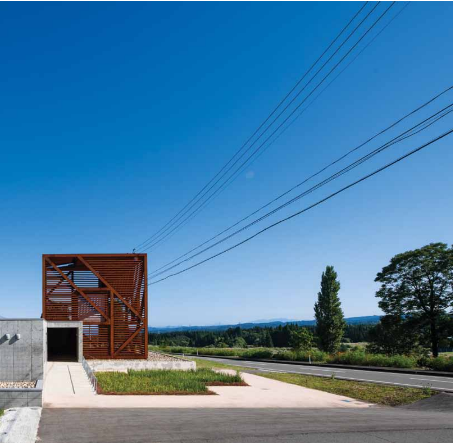
View from the south
