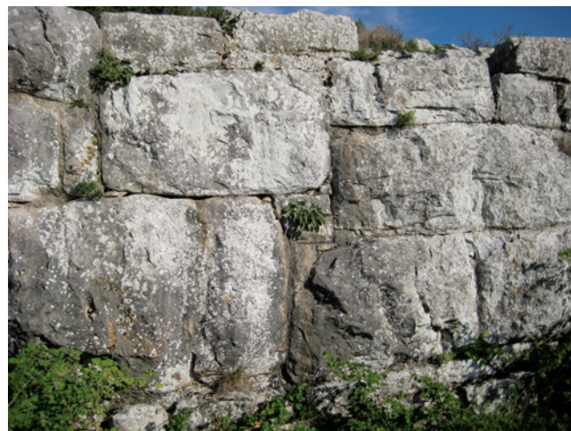
Slika 4. Tehnika gradnje zapadnoga bedema Figure 4. Technique used for construction of western wall
