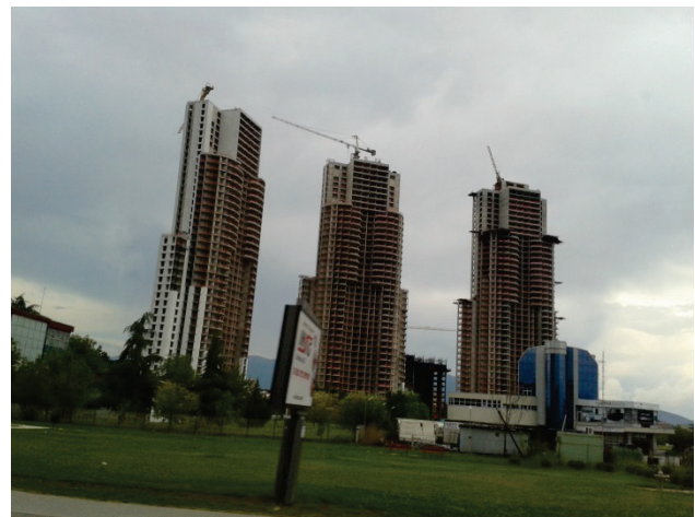
Figure 11 Photos from the construction phase (contd.)
