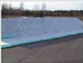
Platna prekrivaju prednji dio pregrade Canvas covering the front of the barrier
