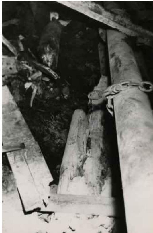
Figure 4. Collapse of roofing within the mine
