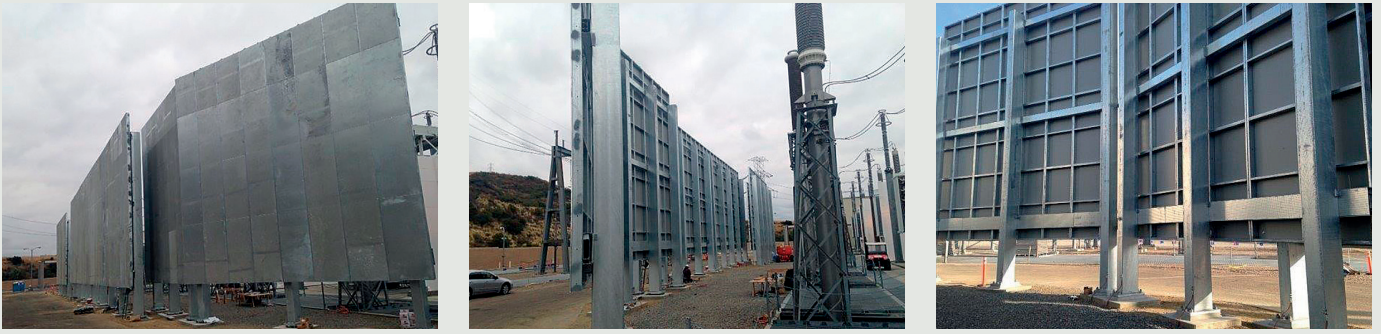
Figure 2. UL 752 tested ballistic fire barriers installed to NFPA 851
