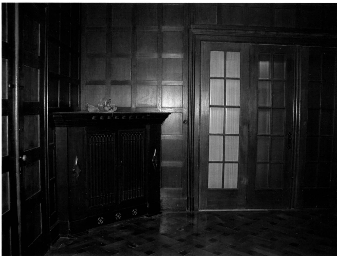
Hall, drveni ormarić za radijator, detalj / Hall, wooden radiator closet, detail
