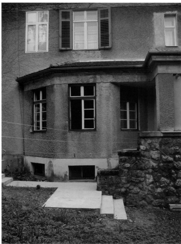
Pogled na erker, blagovaonica / View of the jetty, dining-room
