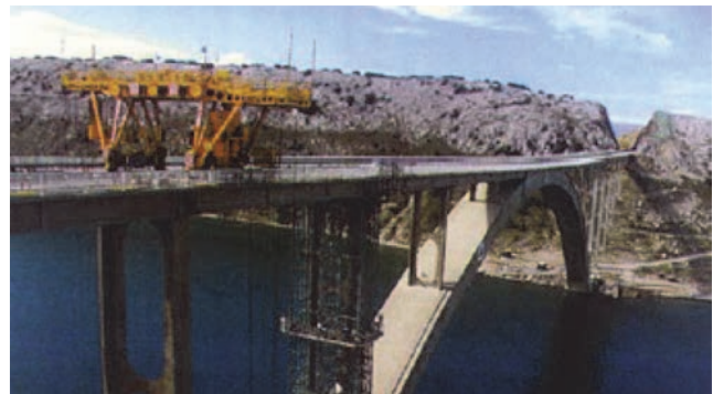
Figure 7. Load relieving scaffold at pier S26 [4]
