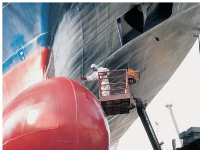
Figure 6 Application of final AF coat in dock, Shipyard Viktor Lenac, Rijeka
